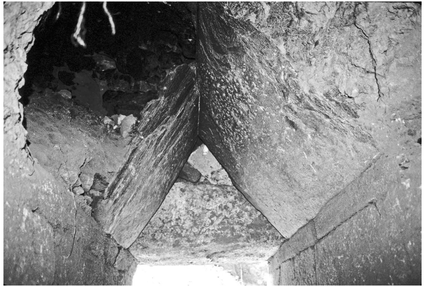
FIG. 6. View of end of dromos during excavation in 1999. Note the reused material sealing the triangular gap between the lintel and the slabs of the pitched ceiling.
